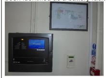
Following a recent fire alarm actuation it was discovered that Zone 12 is not marked on the zone plan. This is being rectified in the near future, monitor.
